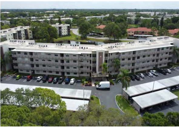
1 Front of Building
