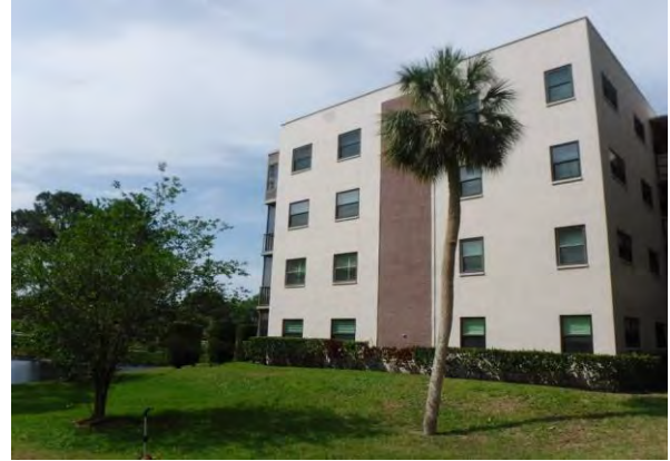
4 Left Side of Building
