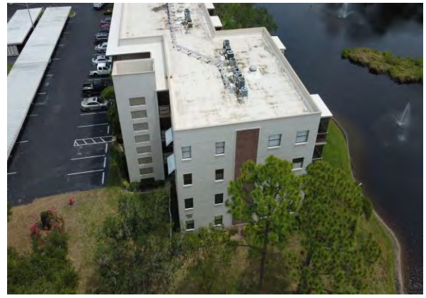
2 Right Side of Building
